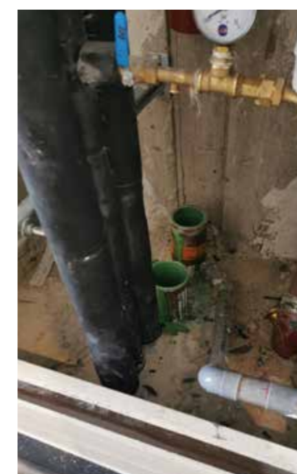
Lining of stag pipes from the top floor
