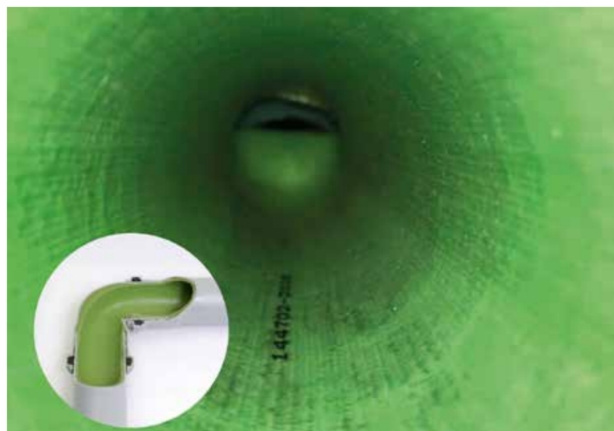
Pipe rehabilitation BRAWOLINER® DN 50
