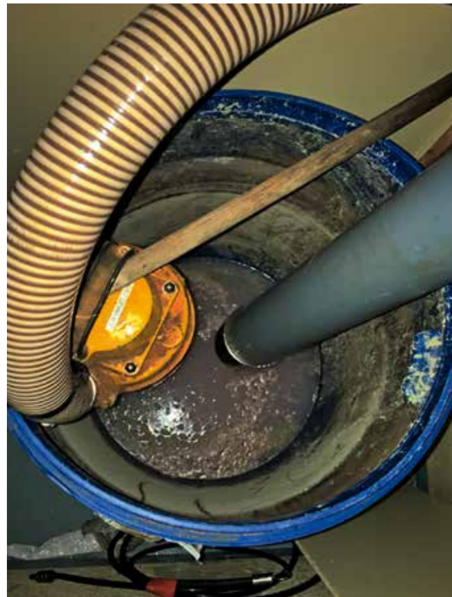
Figure 8 and 8a: Collecting the solids when cleaning the drainage systems
