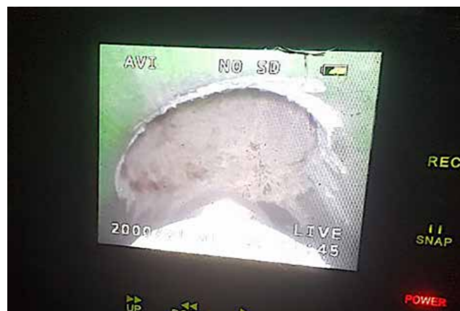
DN 100 inlet opened from a DN 125 downpipe with the cutting robot
