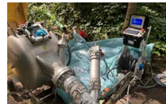
Curing process with the BRAWO® Magnavity
