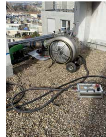
Control of the inversion with the BRAWO® Control Box
