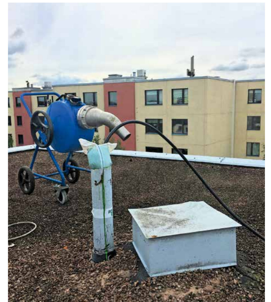
Figure 10: BRAWOLINER® inversion of a downpipe from the roof to the basement
