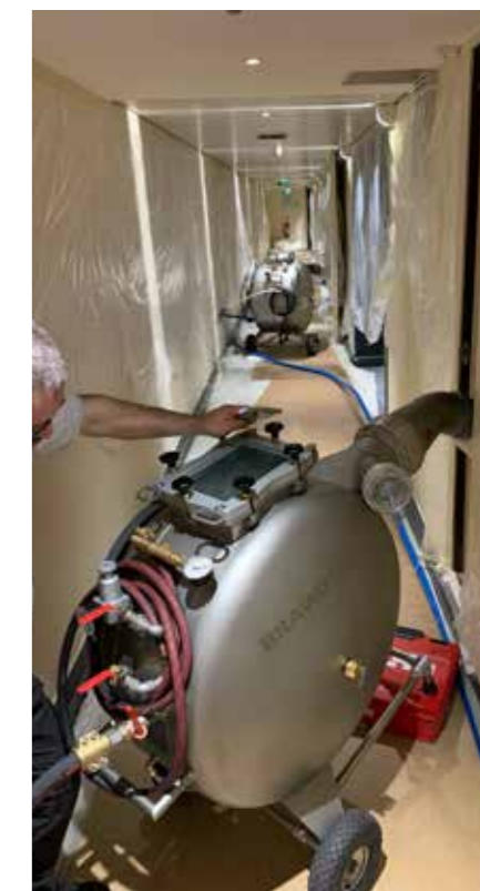
Three installations at the same time
