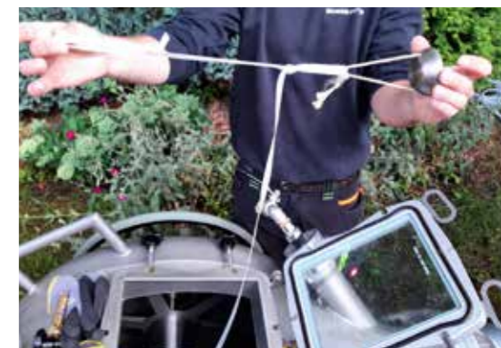
The steel cap enables decoupling of the MEGA LED head at the liner end
