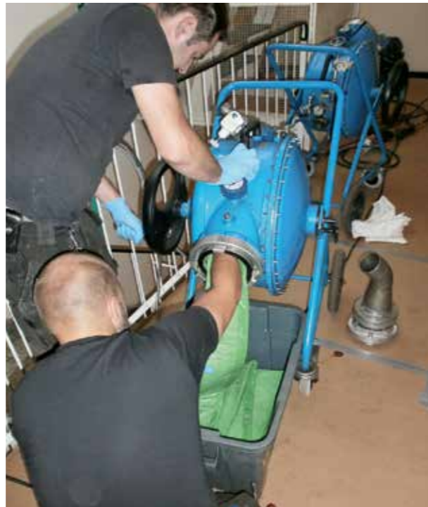
Figure 11: Liner inversion in the nominal diameter range DN 50 to DN 70 with a „liner gun“
