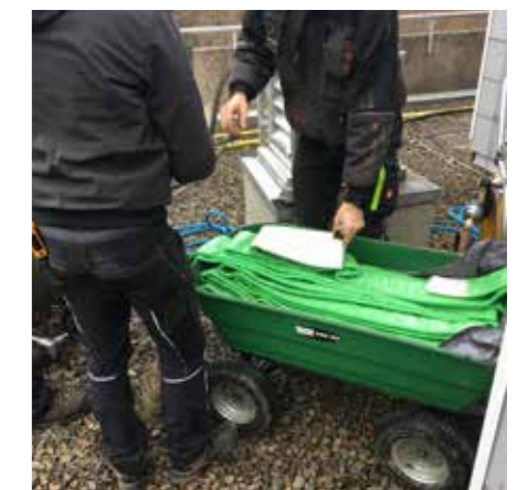
Transporting the hose liner onto the roof
