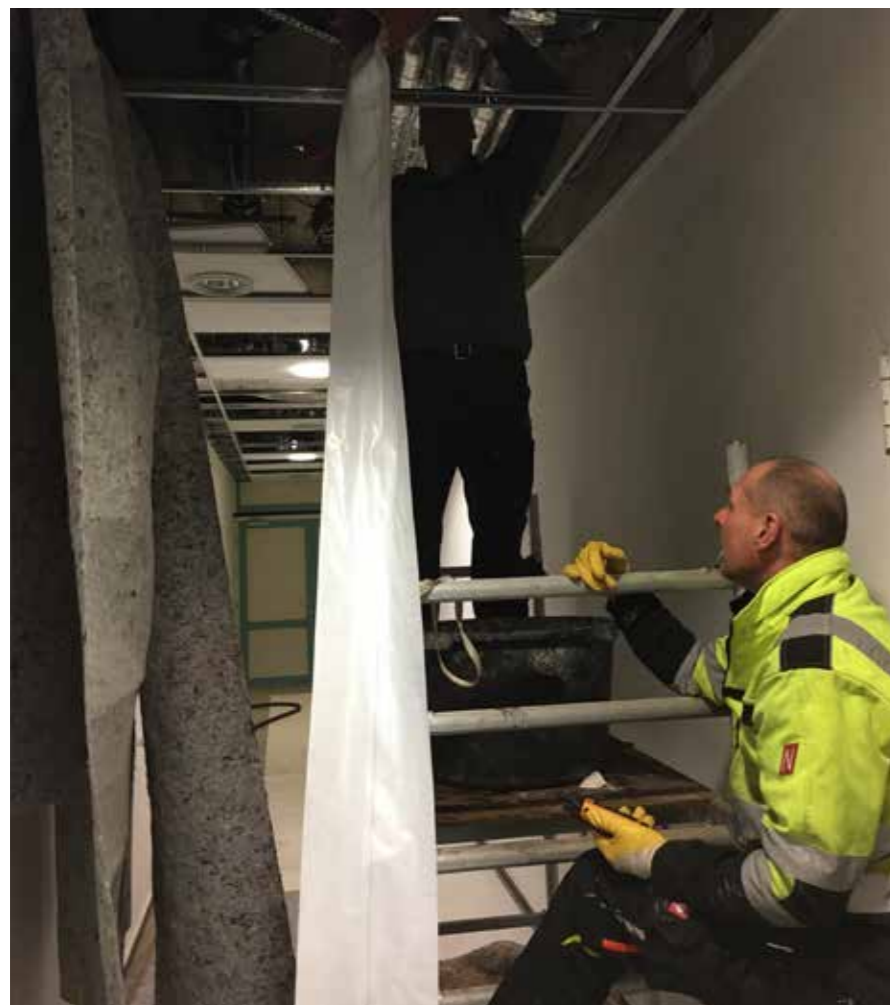
Hose liner arrived at the inversion end on the bottom floor
