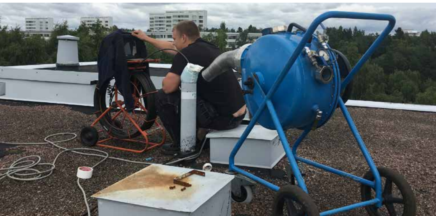
Figure 1: BRAWOLINER® rehabilitation of downpipes above the roofs of Helsinki
