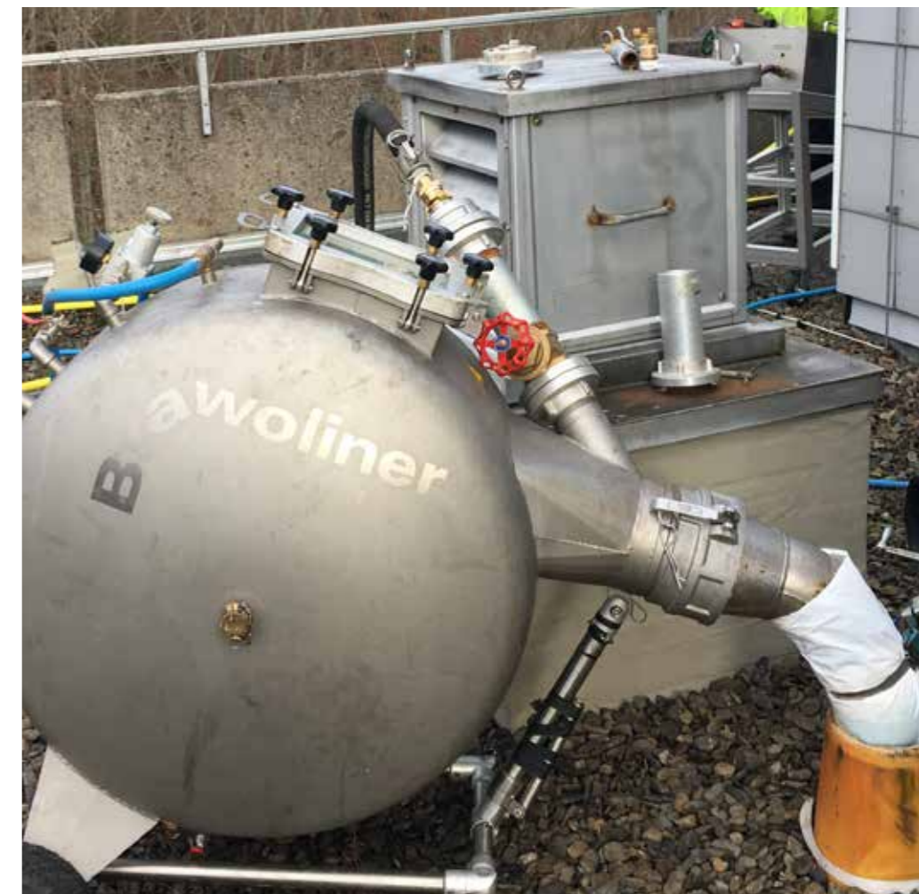
Steam curing the hose liner
