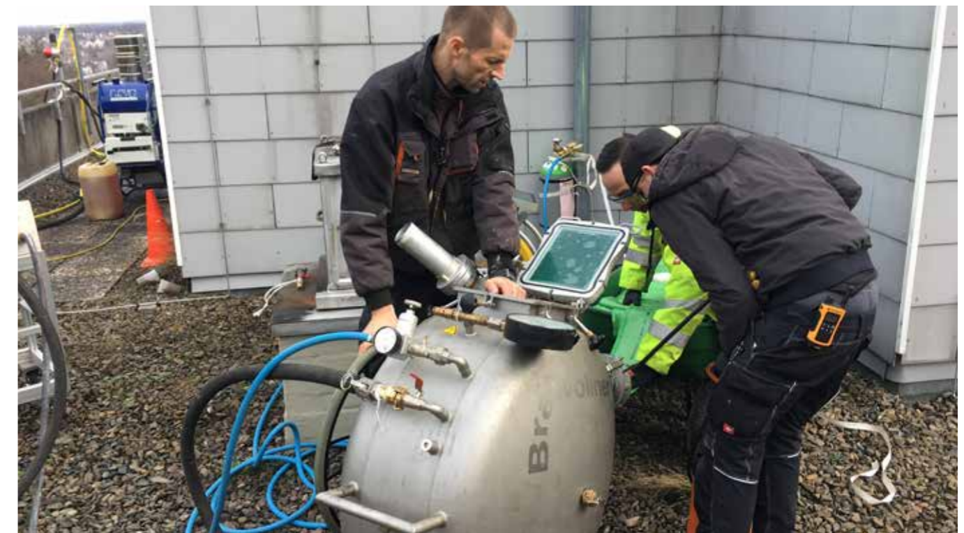
Inversion of the hose liner from the roof
