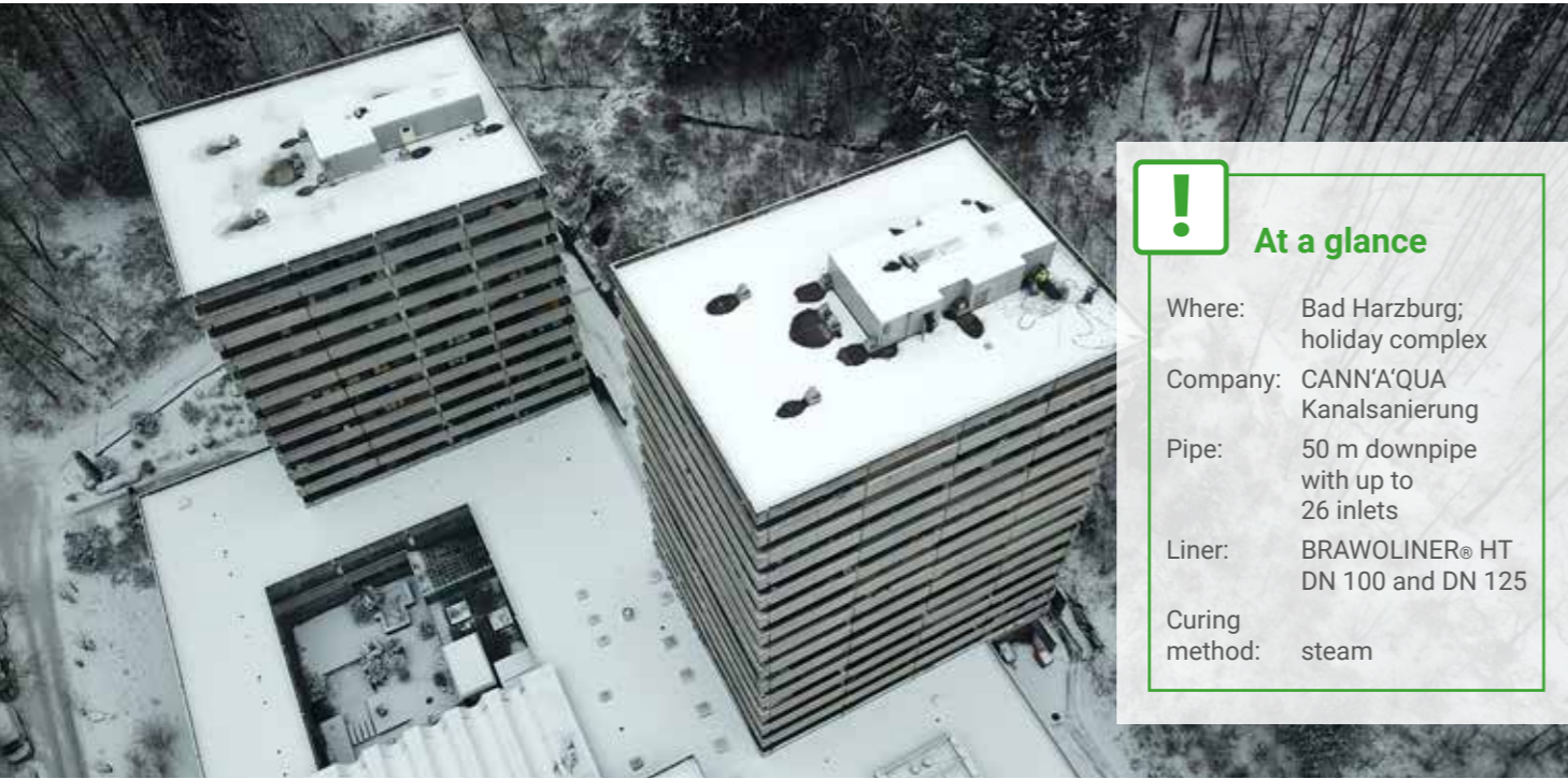
CANN'A'QUA Kanalsanierung for rehabilitating downpipes above the rooftops of Bad Harzburg
