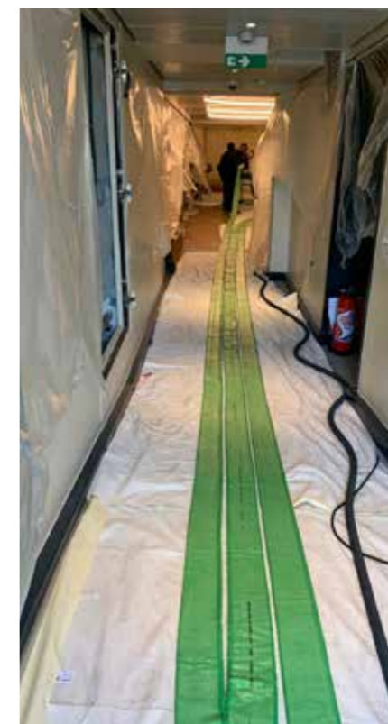
Impregnation of the 70 metres of BRAWOLINER®
