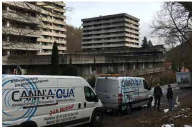
CANN'A'QUA Kanalsanierung from Bad Harzburg in action
